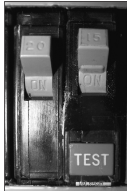
Ground Fault Circuit Interrupter (GFCI) circuit breaker
